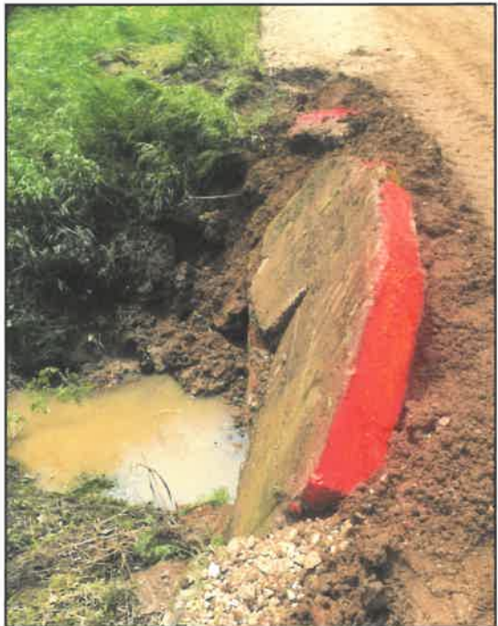
Box culvert on County Road 521
